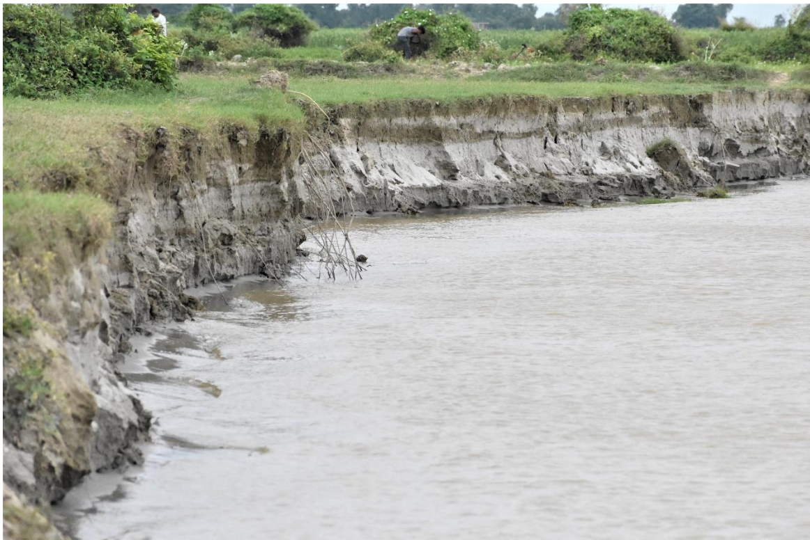
Image 43 : Erosion Prone Bank As Observed Near Jigni Village
