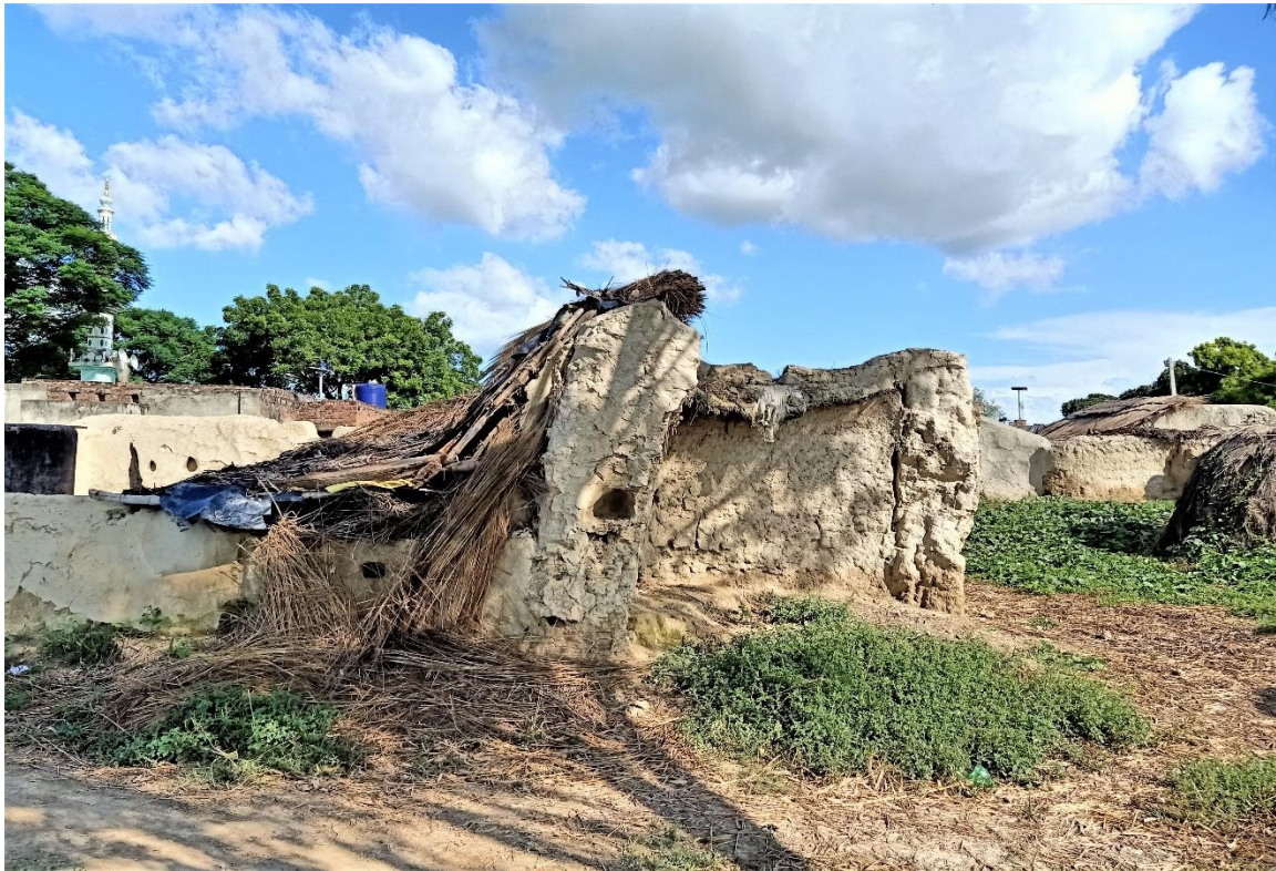
Image 13 : Dried Saccharum Grass Used For Thatching Roof On A Mud House As Observed In Murwa Shaha Buddinpur Village
